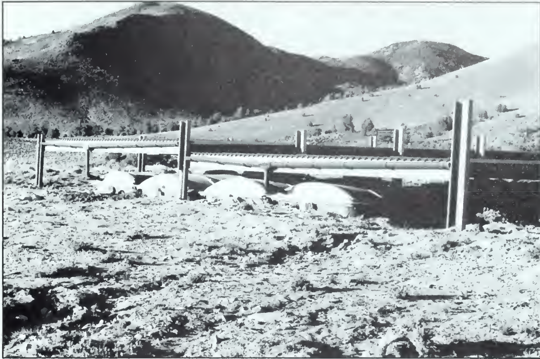
Photo 8. Guzzler showing 16-foot x 32-foot one-unit aprons; shared uprights between aprons; buried tanks, gutter hookups.
